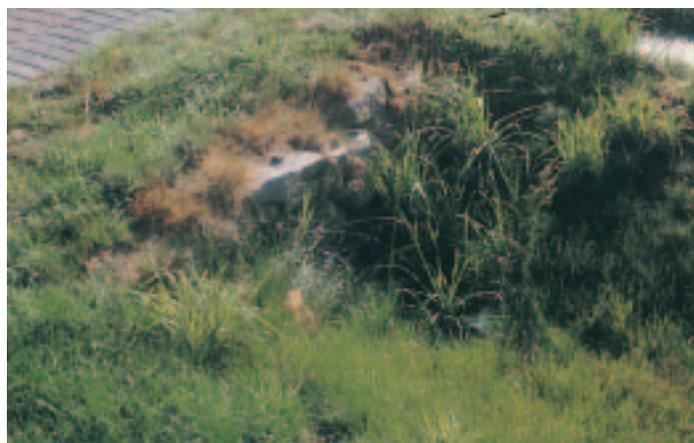
Figure 3. Grass swales rather than curb and gutters enable water to infiltrate and reduce the erosive effects from rapid discharges into streams.
