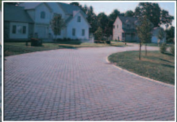
Runoff is being monitored from over 15,000 sf (1500 m<sup>2</sup>) of permeable interlocking concrete pavement in the road and driveways of the Glen Book Green Subdivision in Waterford, Connecticut.
